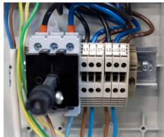
**External Capacitor Power Wiring**
